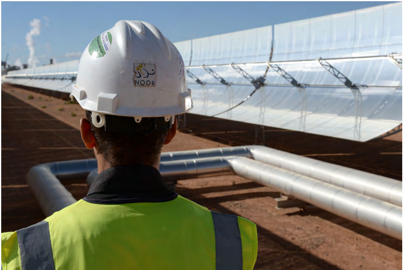
Photo above: A worker standing in front of solar mirrors at the Noor 1 Concentrated Solar Power plant, some 20 km outside of Ouarzazate, Morocco, on Oct. 17, 2015. Photo by Fadel Senna/AFP via Getty Images.
