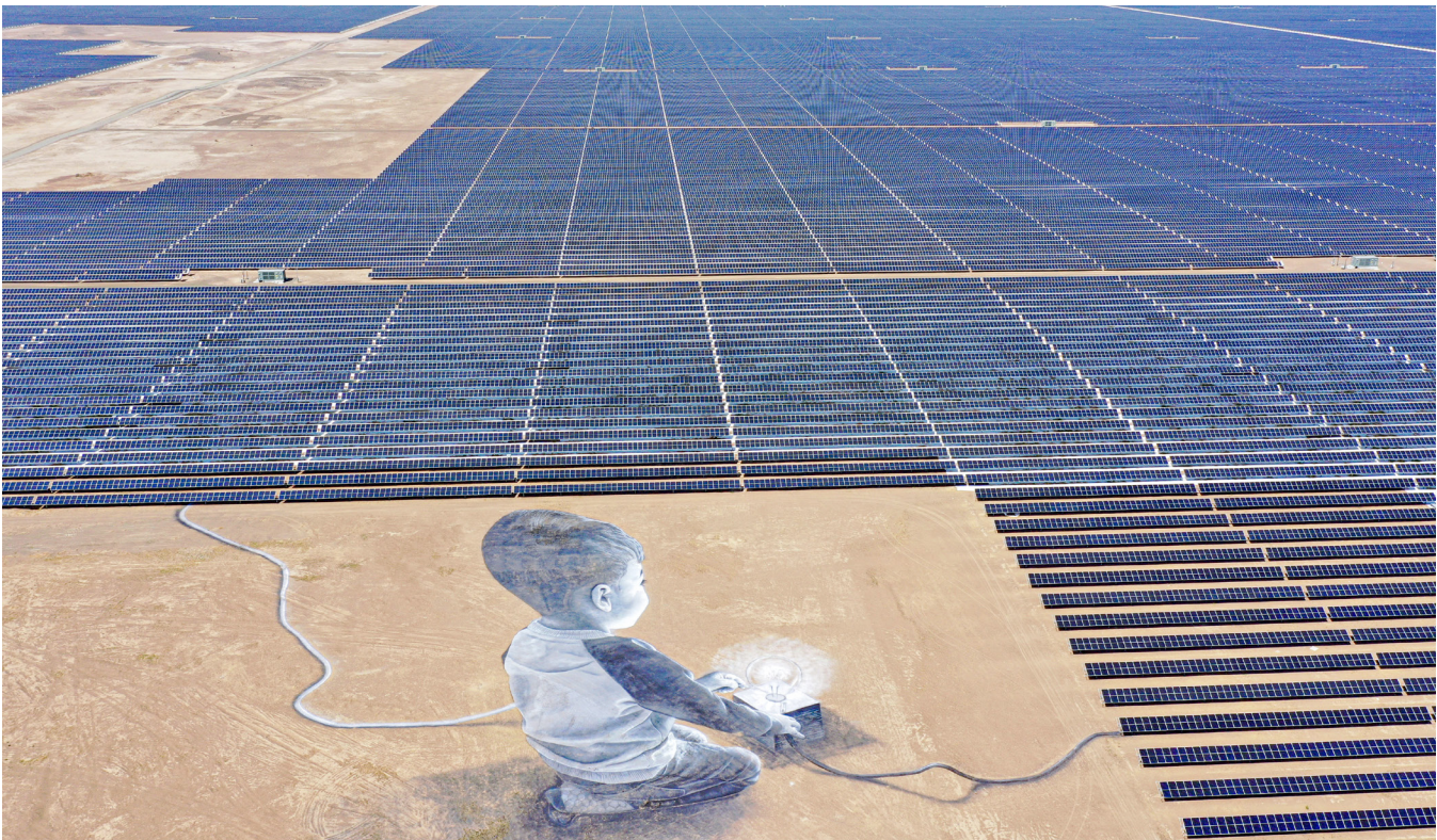
Photo above: An aerial view of the 500,000-panel Ibra solar facility in Ad-Dhahirah, Oman, on April 12, 2023. Photo by Ahmed Abd Alkawayf/Anadolu Agency via Getty Images.
