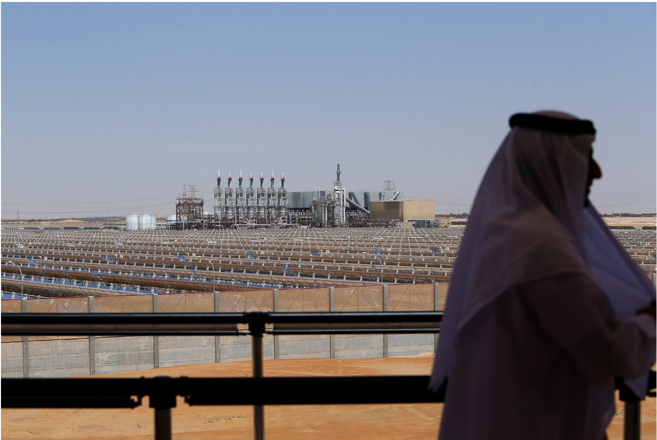
Photo above: An Emirati man stands on a balcony overlooking the Shams 1 concentrated solar power plant in al-Gharibiyah district on the outskirts of Abu Dhabi during the facility's inauguration in March 2013. Photo by MARWAN NAAMANI/AFP via Getty Images.
