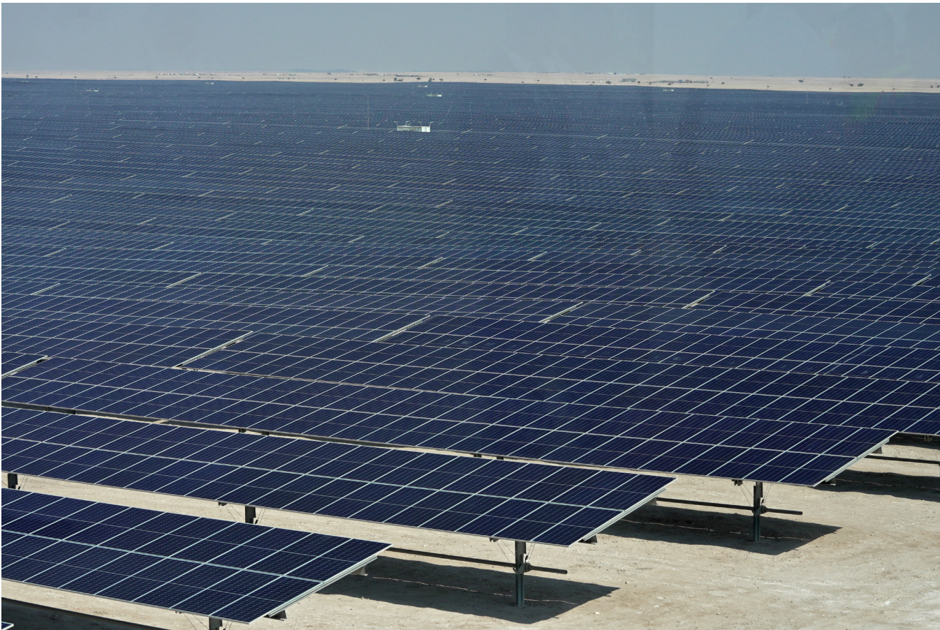
Photo above: Solar panels at the newly inaugurated al-Kharsaah solar power plant in Qatar. Photo by IVAN PISARENKO/AFP via Getty Images.
