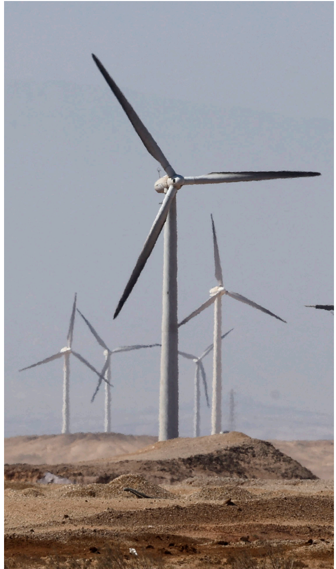
Photo above: Windmills at Zaafarana wind farm south of Suez, Egypt. Photo by Khaled Desouki/AFP via Getty Images.
