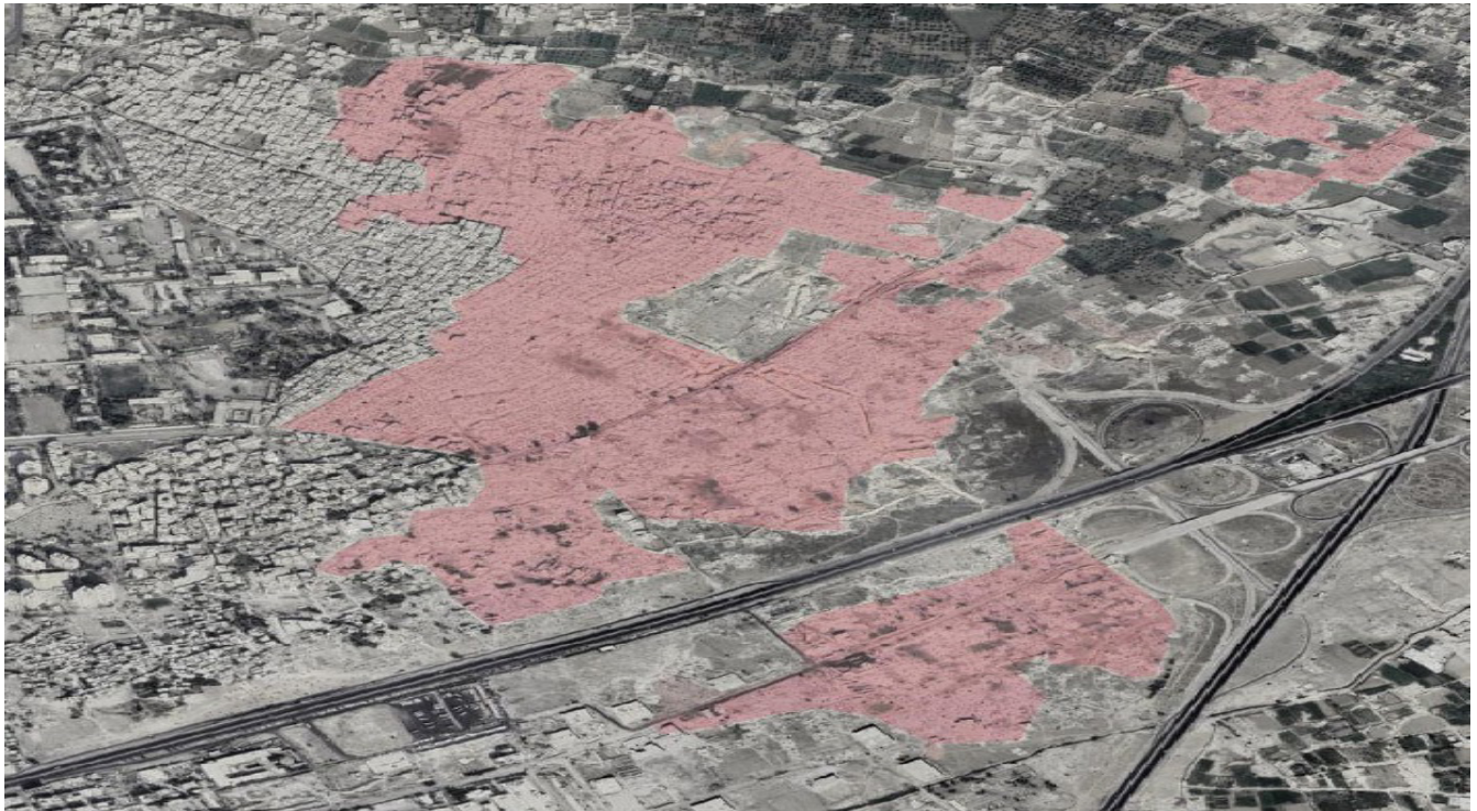
Photo above: Satellite image of Qabun and Tishrine illustrating areas targeted by demolition activities. Source: Google Satellite (2023).
