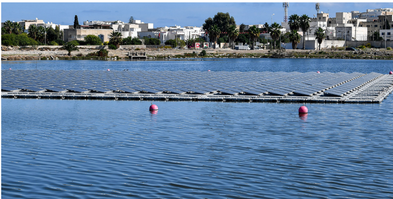
Photo above: Floating solar panels in a water reservoir in Le Kram, on the eastern edge of Tunisia's capital, Tunis. Photo by FETHI BELAID/AFP via Getty Images.
