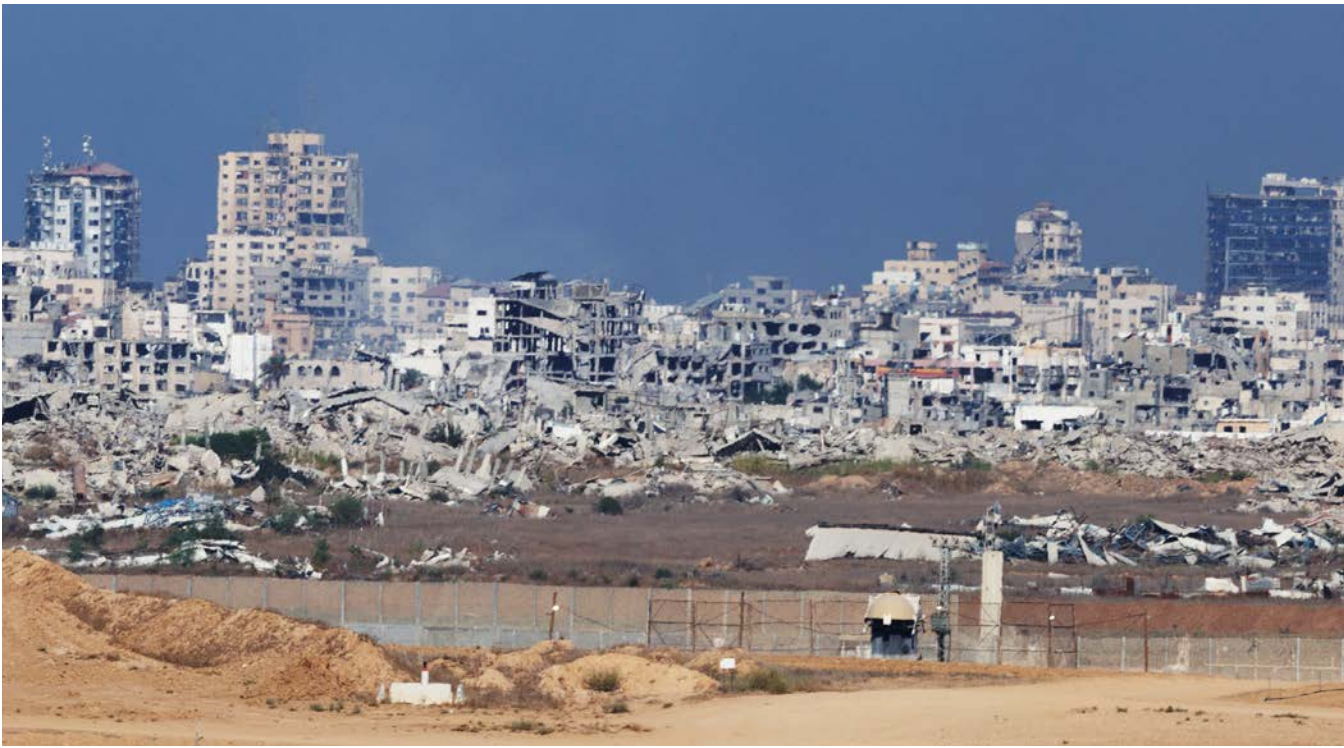
Photo above: Gaza buildings destroyed by Israel during the war with Hamas, October 7, 2025. Photo by Kobi Wolf/Bloomberg via Getty Images.
